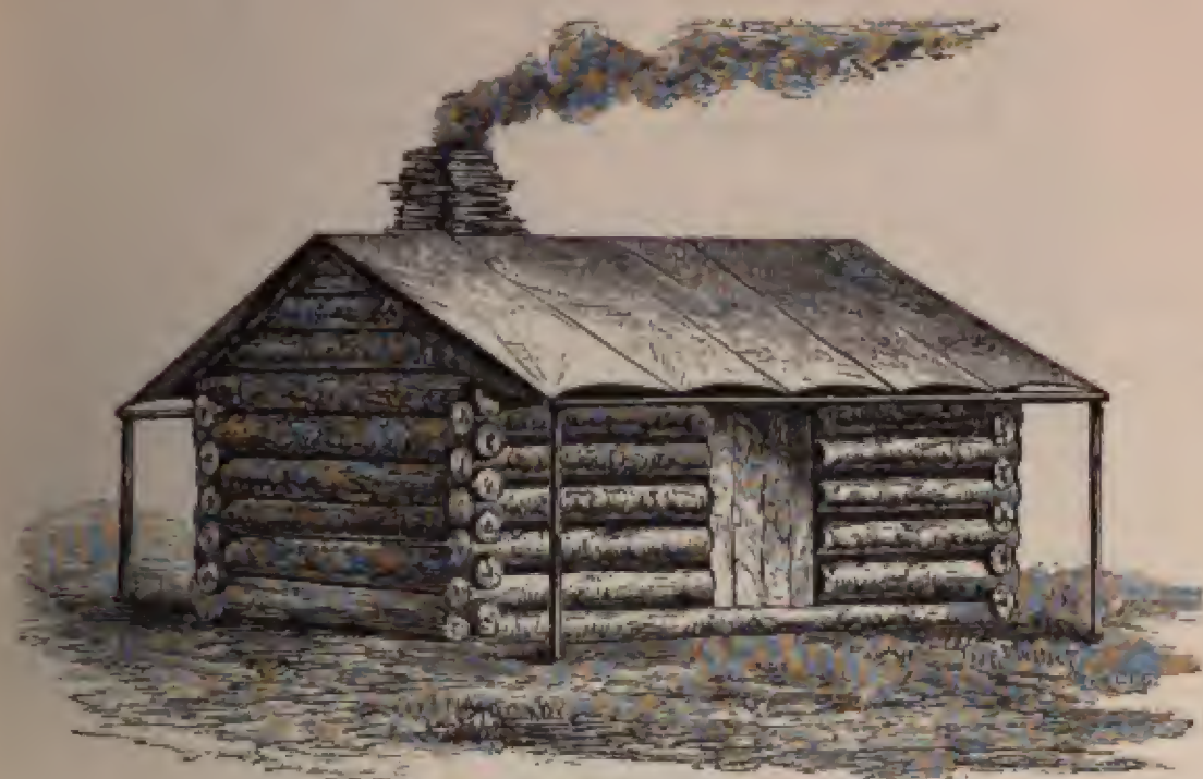
FIG. 197.—Log hut with canvas roof. ( Smart. )
